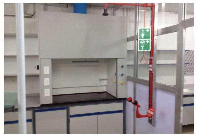
**FFFC** standard widths, External/Internal (mm): 1300/1000, 1500/1200, 1800/1500, 2100/1800, 2300/2000. Depth, External/Internal (mm): 990/650 Height: 2435mm with optional steel support frame (+optional infill panel)
