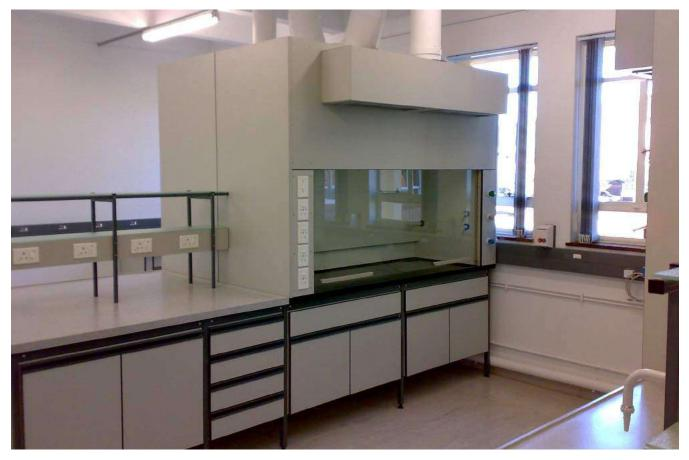
Supply air ducting & remote add air fan will be required. Auxiliary Air hoods are based on a 50% supply air to make up for room supply deficiency.
