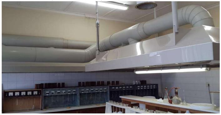
Canopy hoods can be fitted with additional side panels to further isolate the extraction area.
